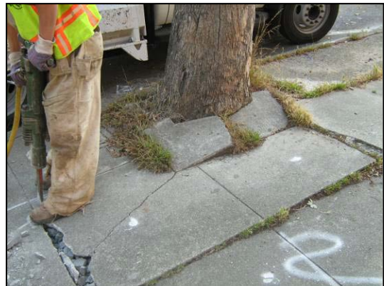
Cracked and buckled sidewalk
