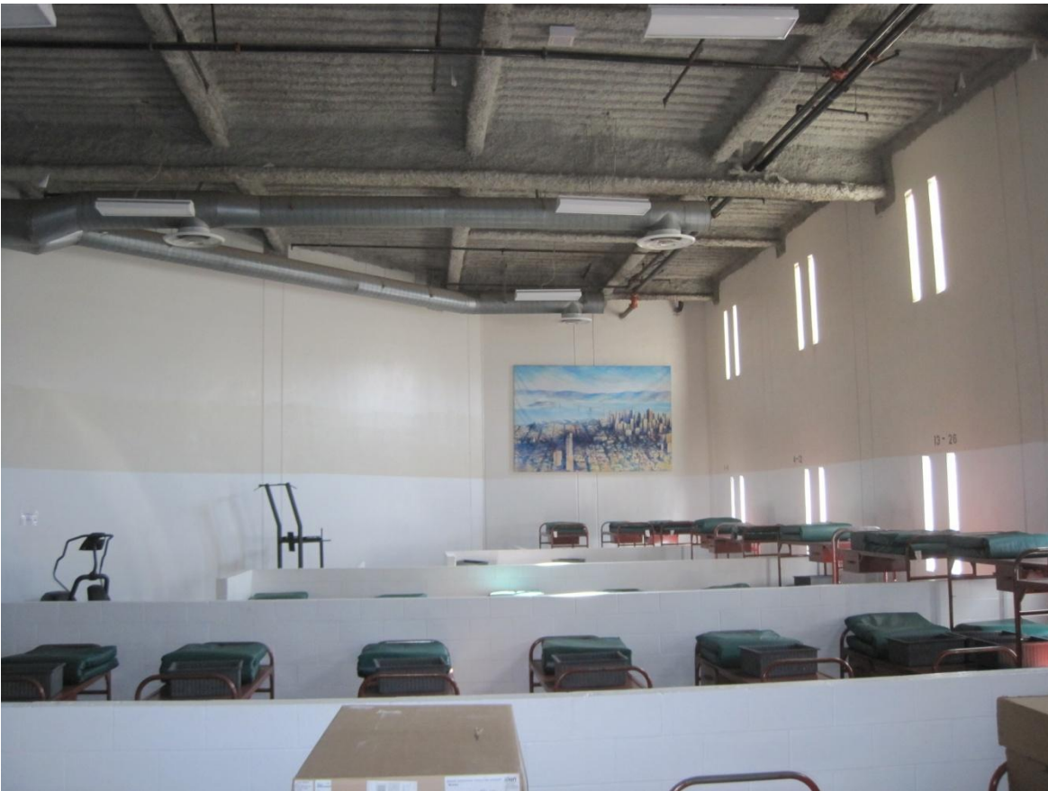
Figure 2 – Typical Interior and Exterior Tilt-up Concrete Walls
