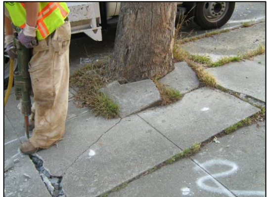
Cracked and buckled sidewalk
