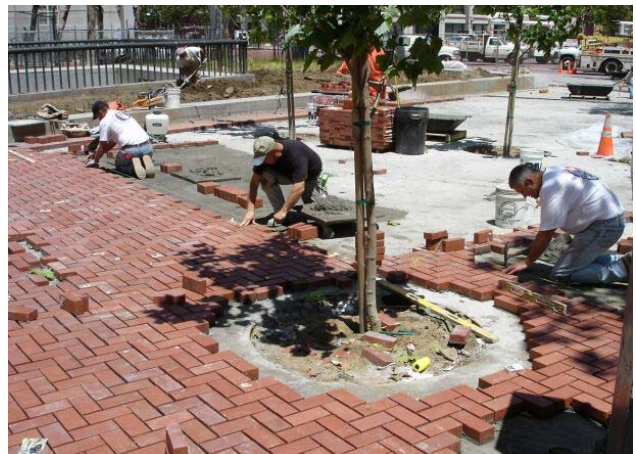
United Nations Plaza Upgrades
