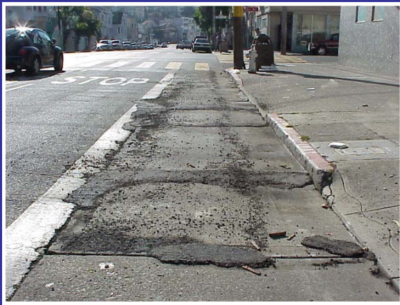
Cracking and Erosion
