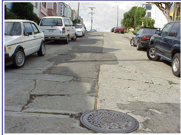
Trenched and broken surface around utilities
