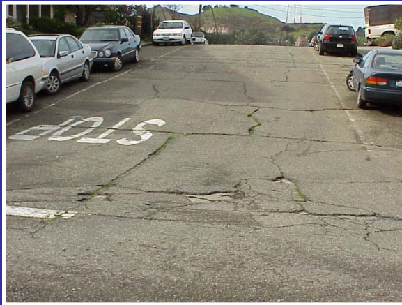
Cracked pavement and potholes
