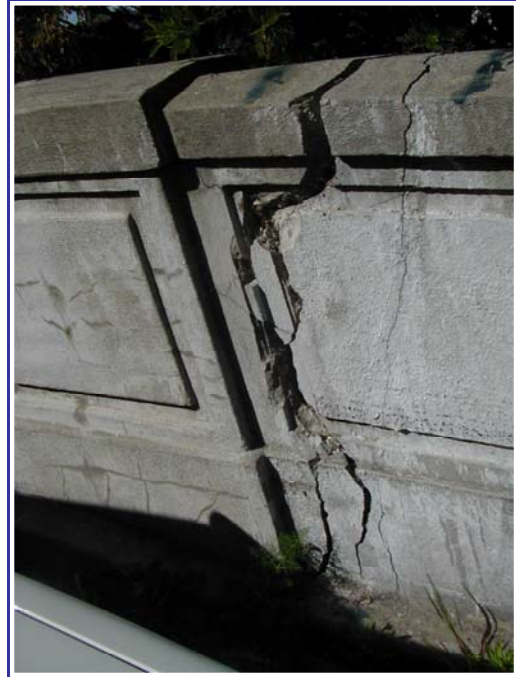
Major cracking of street structure
