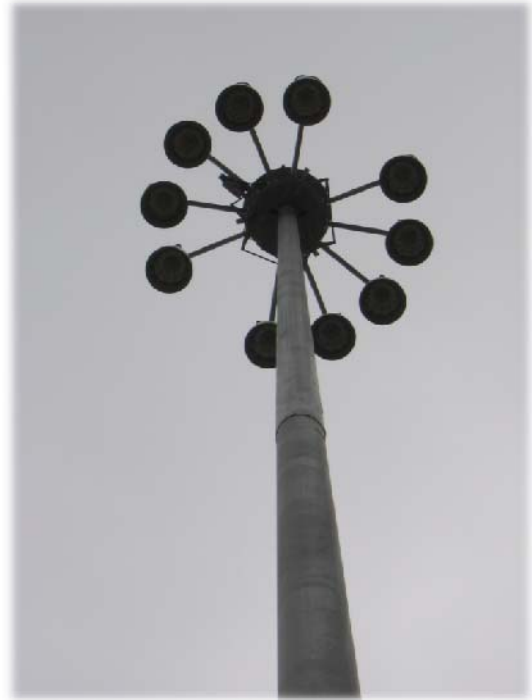
80 Foot High Mast Fixture
