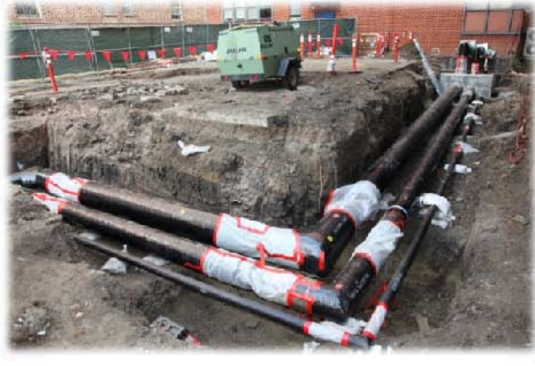
Underground Work at the Hospital Site
