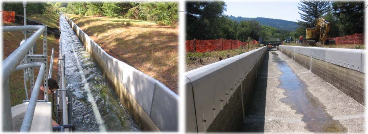
Pulgas Discharge Channel
