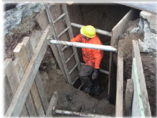
Crew Repairing Sewer
