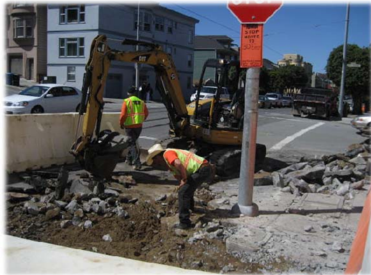
Construction on Fourth Street
