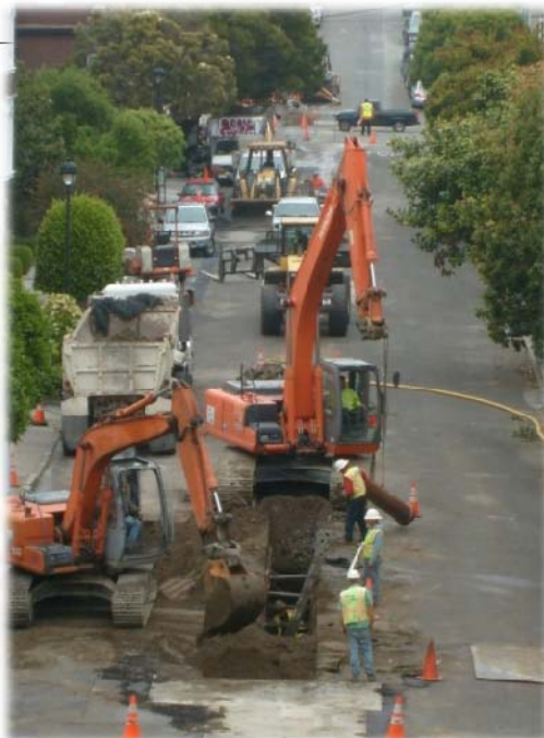
Emergency Sewer Replacement on Vallejo Street
