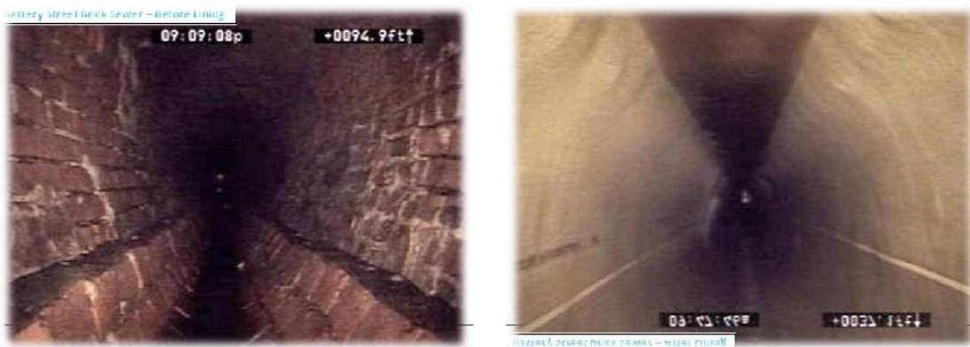
Battery Street Sewer, Before and After Installation of Lining
