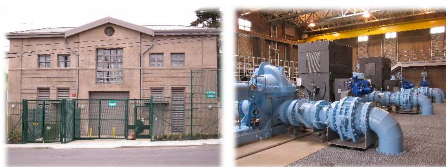
Exterior and Interior of Alemany Pump Station
