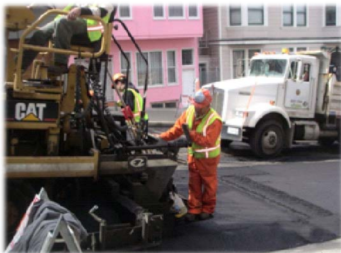
DPW Crew Paving Street
