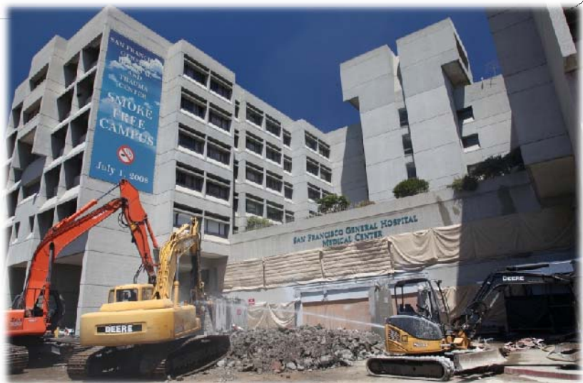
Excavation Begins for the SFGH Rebuild Program
