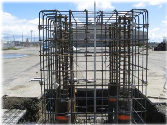
Pier 80 Electrical Site
