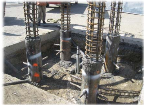
Pier 80 Electrical Site
