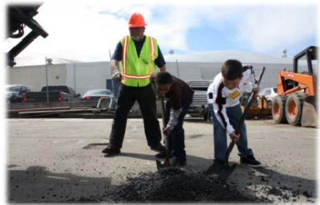
Students Learn How to Fill a Pothole
