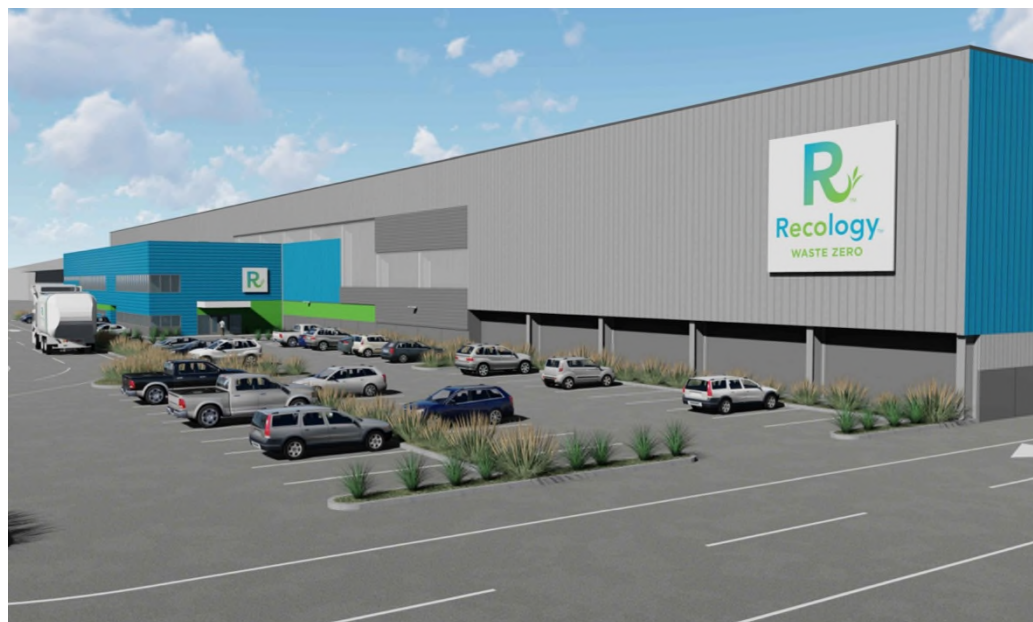
New paving with stormwater improvements
