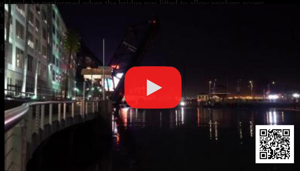
► Passersby may have seen the historic drawbridge raised the night of Jan. 23 so crews could replace corroded bolts – work that could only be performed when the bridge was lifted to give access to workers.
