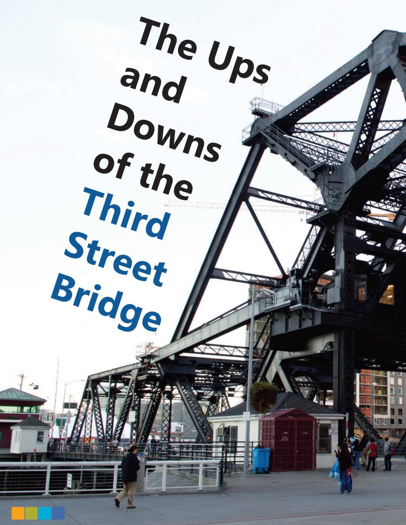
Construction crews completed the first phase of rehabilitation work on the historic Third Street Bridge, which involved preliminary counterweight repairs. ►
