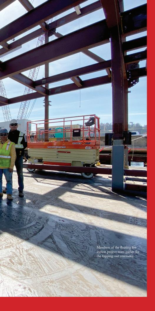
The San Francisco Fire Department's floating station, which is on track for a spring 2021 completion, is being built atop a steel float and anchored by four guide piles, which will allow the structure to rise and fall with the natural tide of the Bay, king tides and anticipated sea-level rise.
