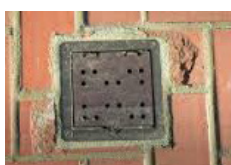
sewer vent cover
