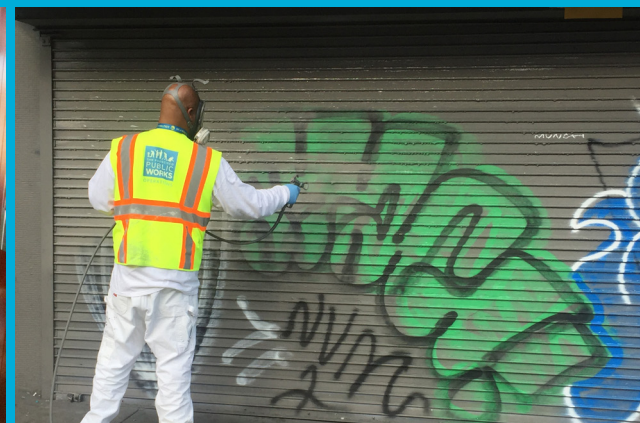
Graffiti paint out
