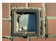
Missing sewer vent cover
