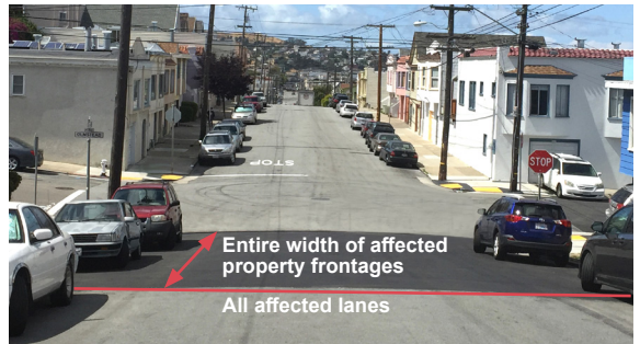
Acceptable/correct paving restoration
