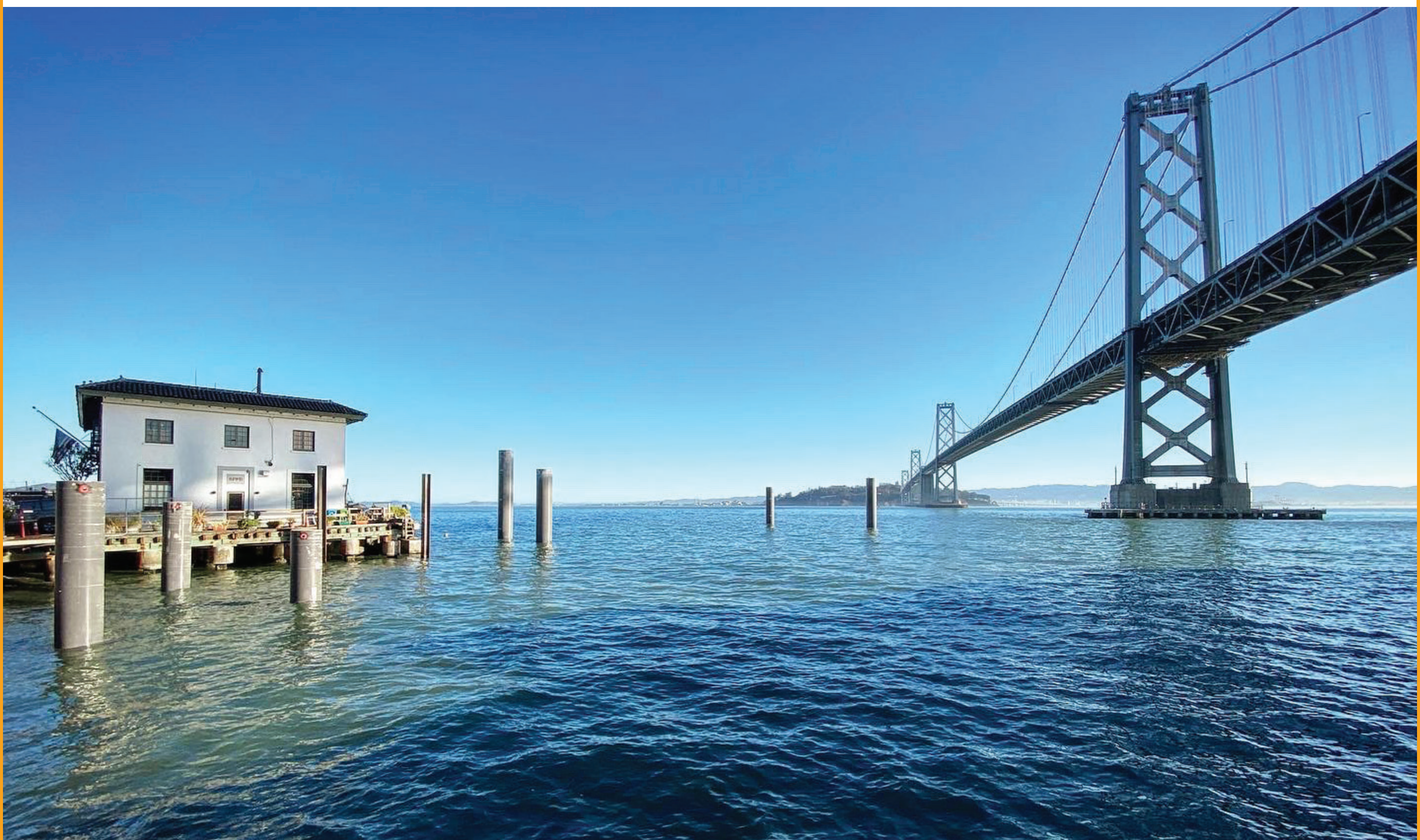
The existing fire station at Pier 22 ½ along The Embarcadero will be replaced with a new structure.
