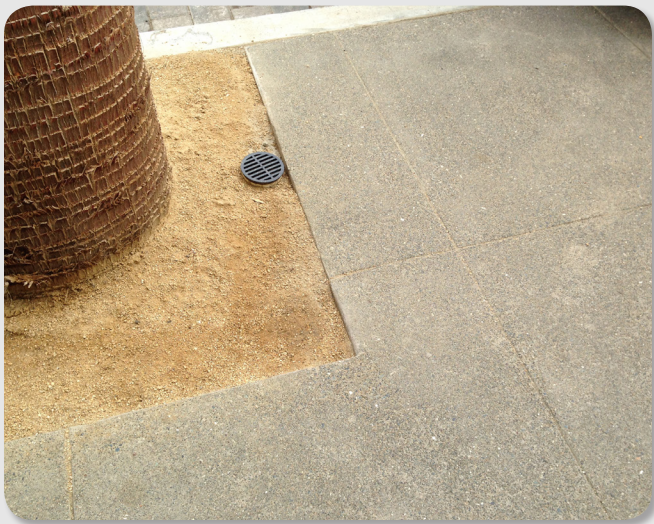
+ CONCRETE SIDEWALKS w/ Integral Color "Mesquite" #677
