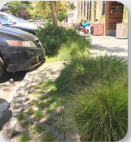
+ TURF BLOCK UNIT PAVERS w/ planting & irrigation reconstructed only at existing locations along 22nd St
