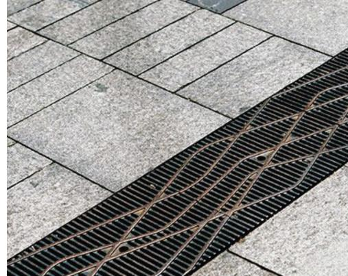
INTEGRAL COLOR CONCRETE STAIRS TRENCH DRAIN CAST IRON GRATE
