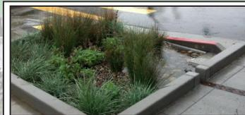
RAIN GARDENS incorporated into bulb-outs capture stormwater runoff from streets, roofs and parking lots. Plants and soil absorb water, reducing the amount of runoff to the sewer system.
