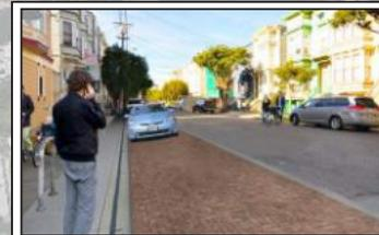
PERMEABLE PAVEMENT enables stormwater to soak through the roadway and into the ground, rather than rapidly flush into the sewer system.
