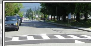
RAISED CROSSWALKS bring the level of the roadway to that of the sidewalk, forcing roadway users to slow down before passing over the crosswalk.
