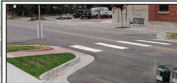
BULB-OUTS extend the sidewalk at intersections, reducing the distance to cross the street and increasing visibility between pedestrians and people in the roadway. Bulb-outs also make corners sharper, ensuring that right-turning bicyclists and motorists take the turn slowly.
