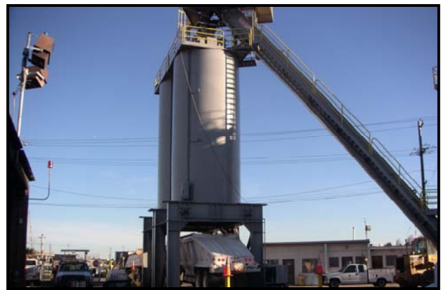
DPW's Municipal Asphalt Plant
