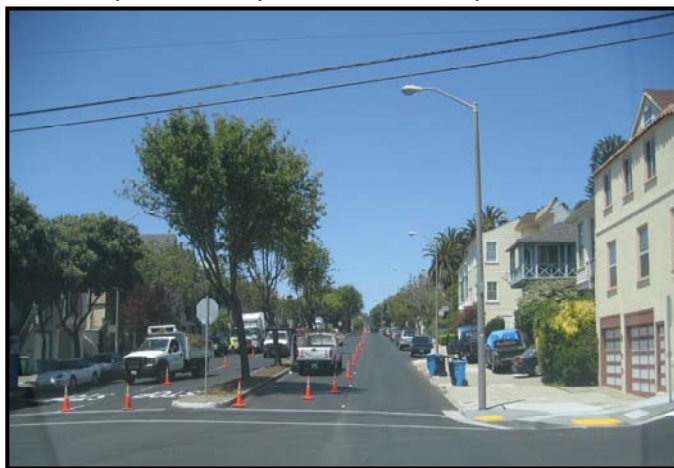
Monterey Boulevard Renovation Project
