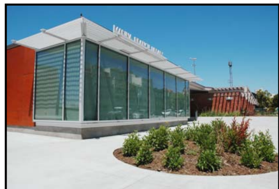
New addition to the Marina Branch Public Library
