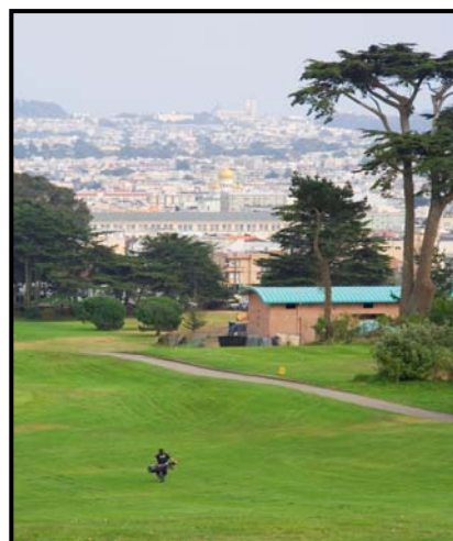
The Lincoln Park Pump Station
