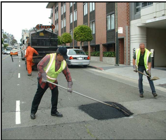
BSSR crew patch paving a street
