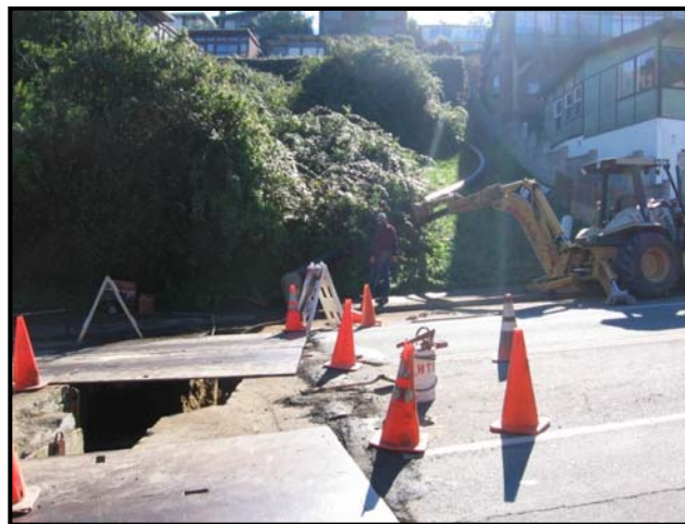
Stanyan Street Emergency Sewer Replacement
