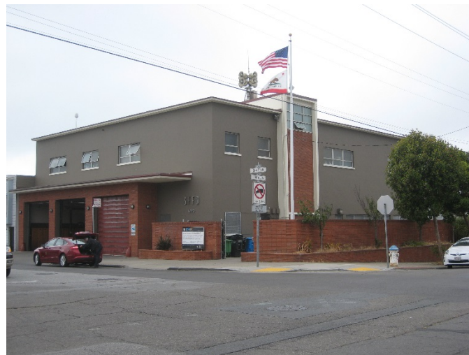
Station 17 – Exterior Envelope
