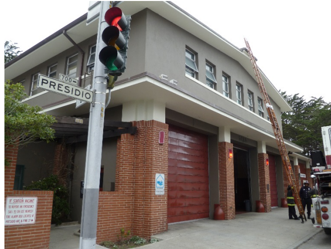
Station 10 – Exterior Envelope
