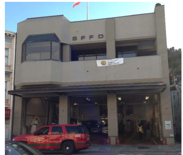
Station 2 – Exterior Envelope
