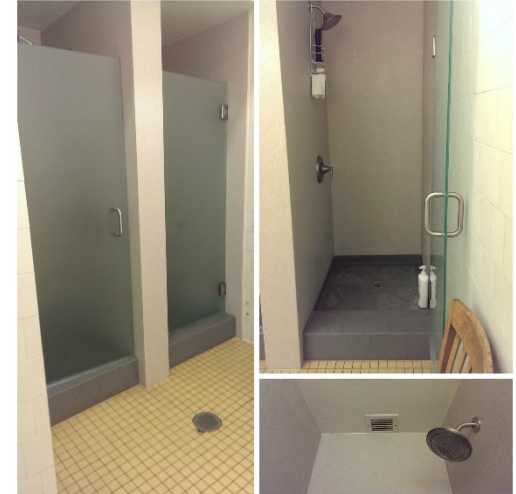
Station 26 – Shower Renovation
