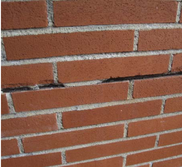
Station 10 Grout Repair
