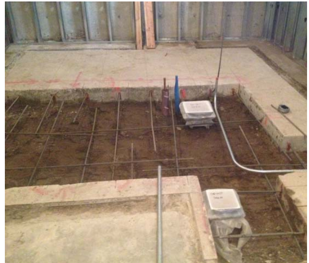
Slab Infill at kitchen
