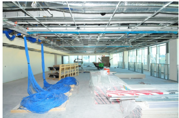
Cabling work at 5 th Floor at West Tower
