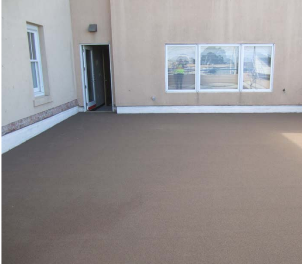
Finish Roof Coating
