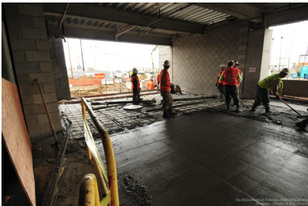
Concrete placement at street level parking
