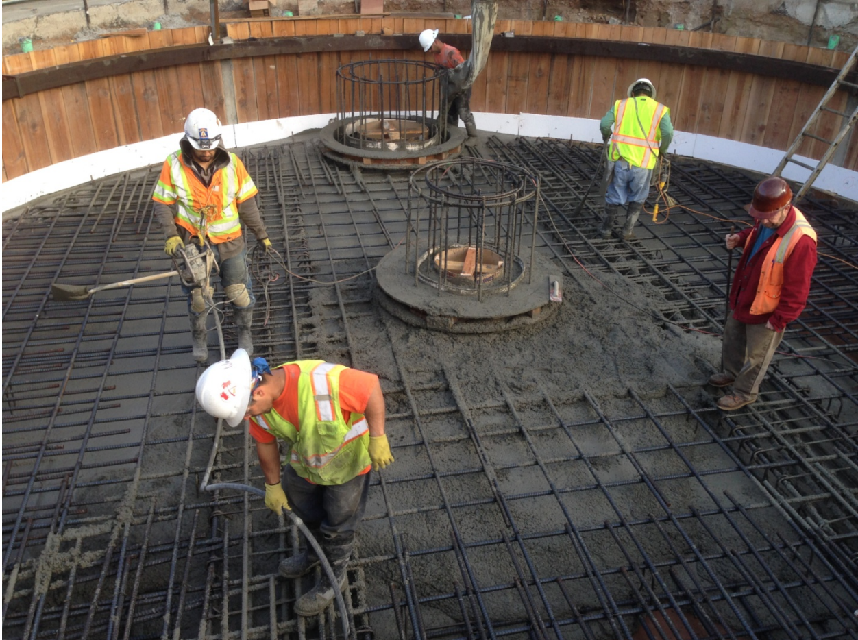
37 th Avenue/Lawton Street Roof of Cistern
