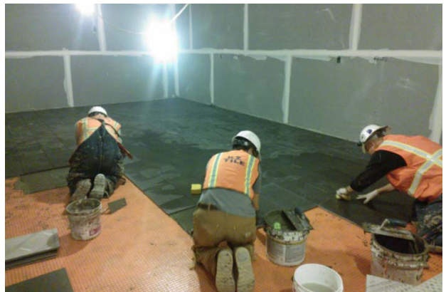
Tiling installation at 3 rd Floor Locker Room
