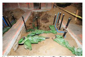
Under-slab utilities installation at Fire Station 30
