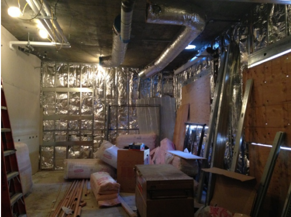
Wall Insulation at Kitchen
