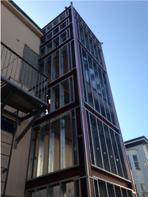
Elevator Wall Framing
