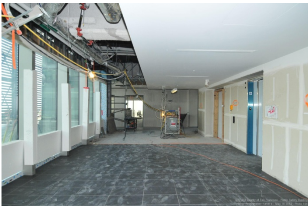
Staff elevator lobby at Level 4
