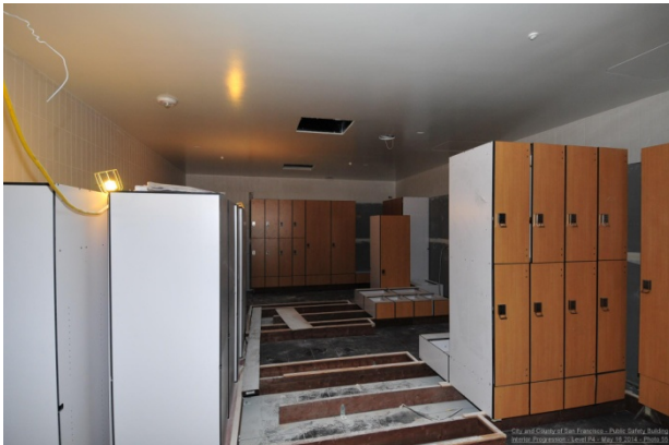
Locker installation at Level 3 Women's locker room
