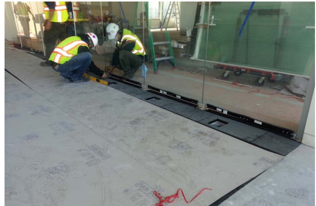
Interior partition installation at L3 HQ fitness area
