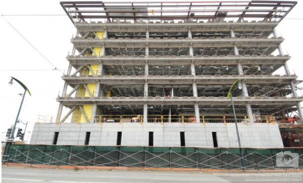
North Elevation of building (along Mission Rock)
