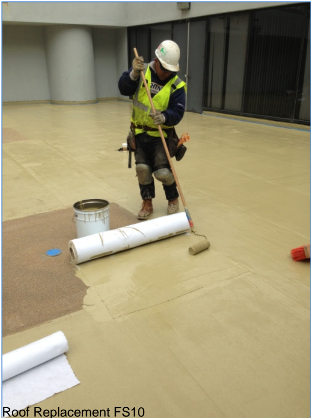
Roof Replacement FS10
