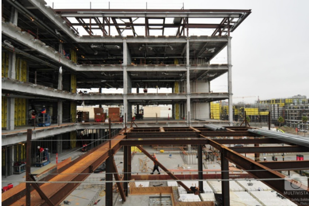
View of West Tower from FS4 Roof (Level 3)
