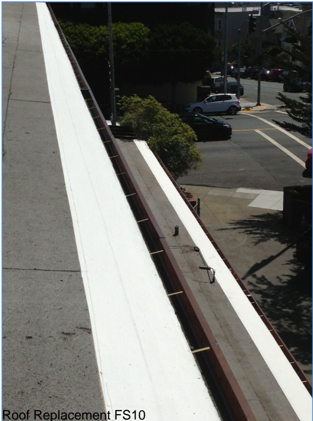
Roof Replacement FS10
