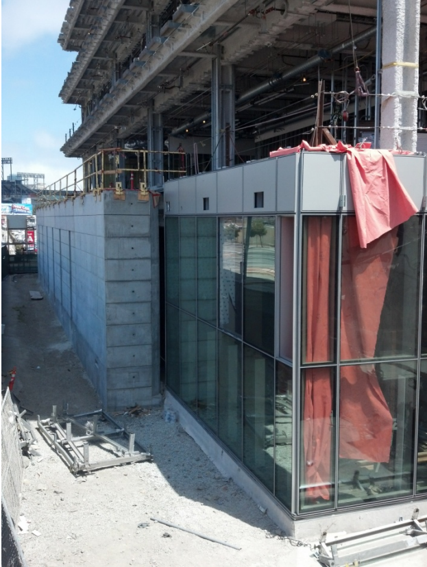
Curtainwall Glazing Assembly at Southwest corner of building
