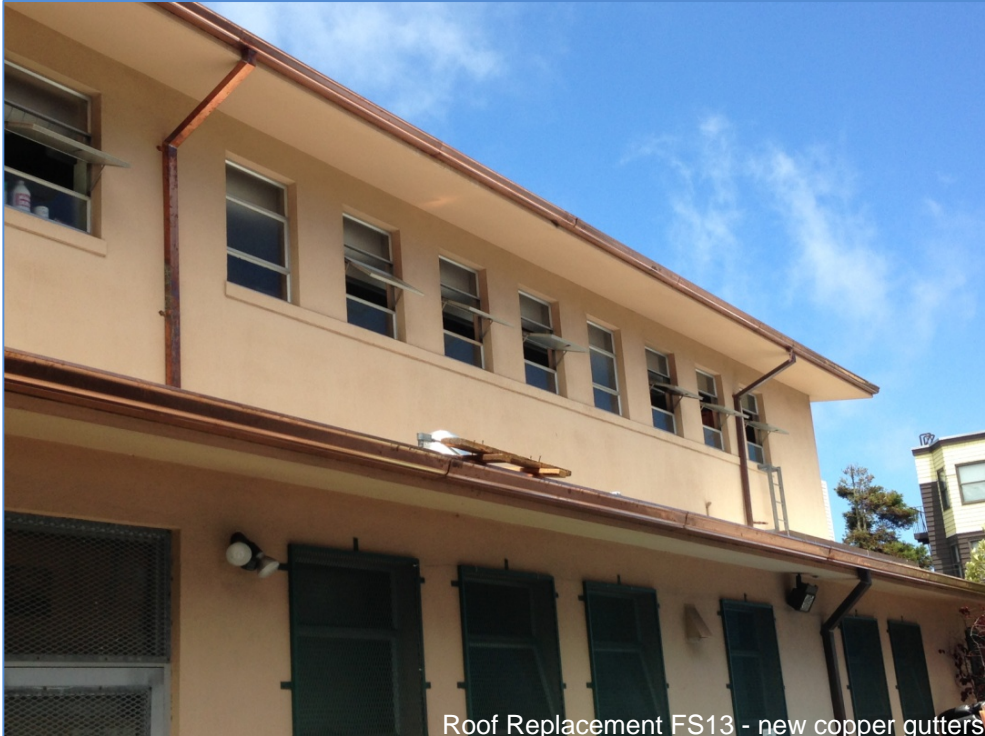
Roof Replacement FS13 - new copper gutters
