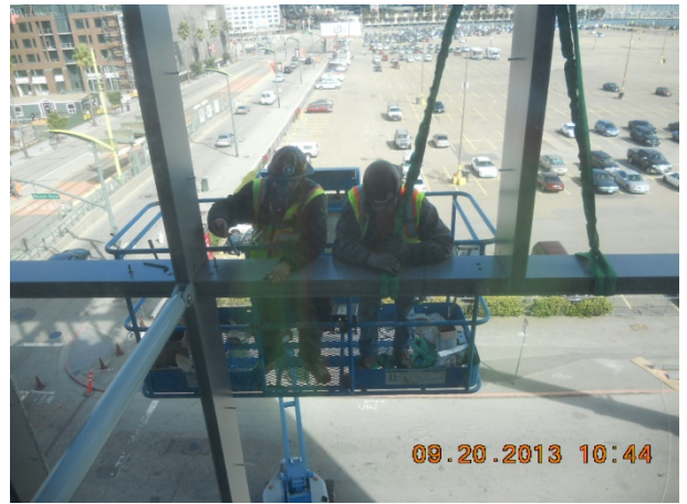
Installation of framing for north building screen
