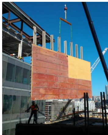
Removal of architectural concrete form
