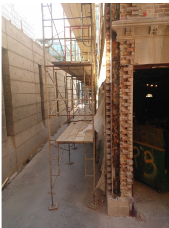
Scaffolding at FS30 for brick repair work
