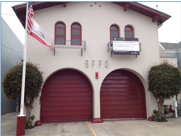
Exterior Envelope Station 40 Painting
