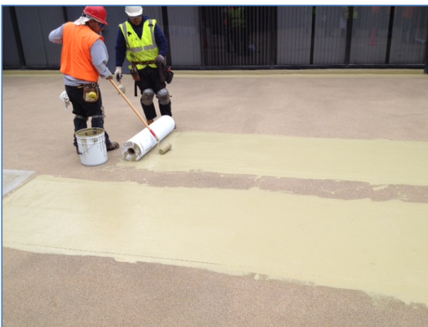
Roof Replacement Station 13 Deck Coating
