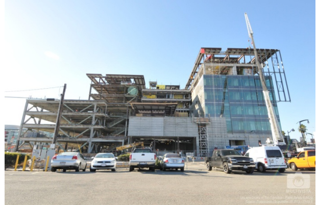
View of North facade
