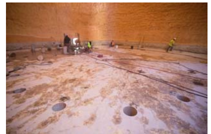
Jones Street Tank
