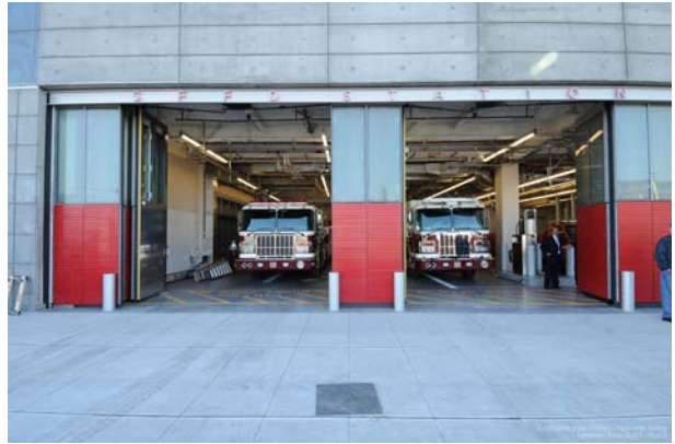
Fire Station no. 4 apparatus bay
