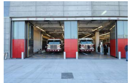
Station 4 Apparatus Bay
