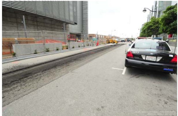
Paving in progress at China Basin Street
