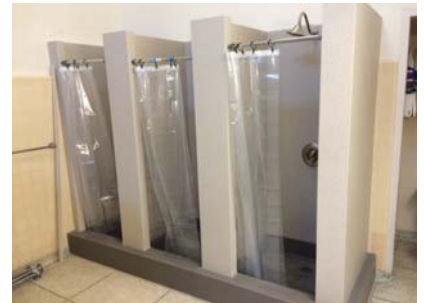
Station 38 Shower Replacement
