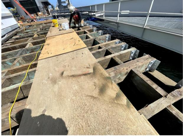
Structural Repairs at North Apron Reconstructed Pile Caps & New Steel Beams & Girders
