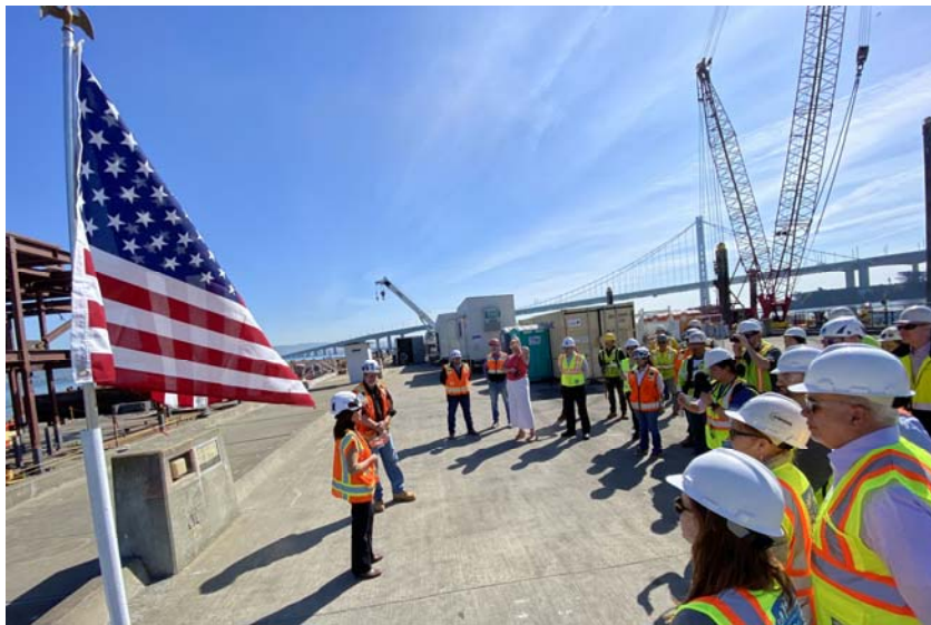
Fireboat Station No. 35 Topping-Out – Erection of Final Steel Beam – March 4, 2020
