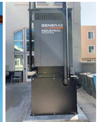
Fire Station 31 Generator Replacement
