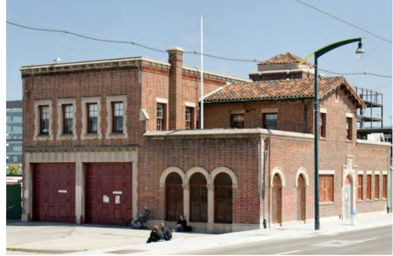
Fire Station #30 on site
