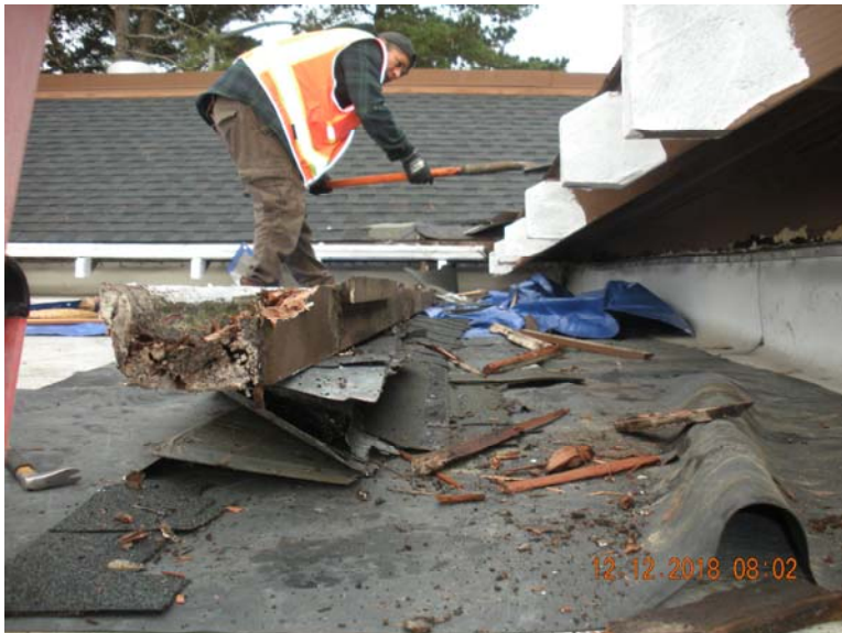
Existing rotted gutters have been demolished; rafter tail replacement is under progress.
