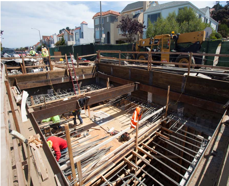
17 th Avenue & Pacheco Street cistern, June 2016
