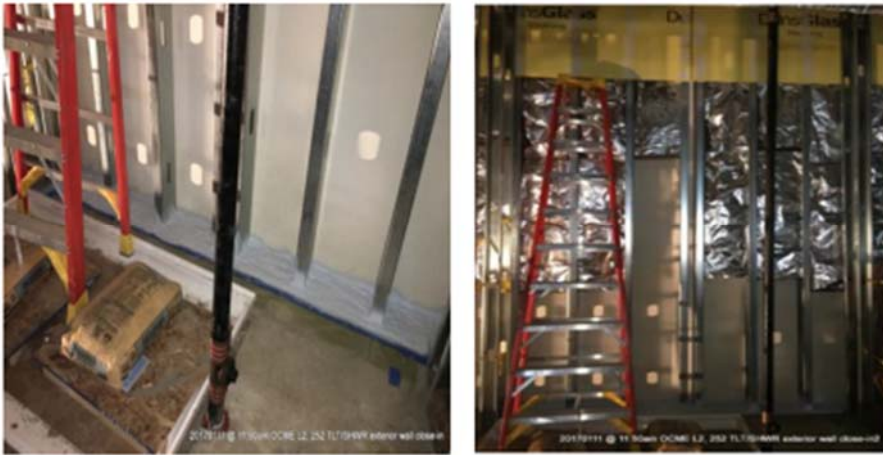
Shower Room 253 exterior wall insulation and close-in.
