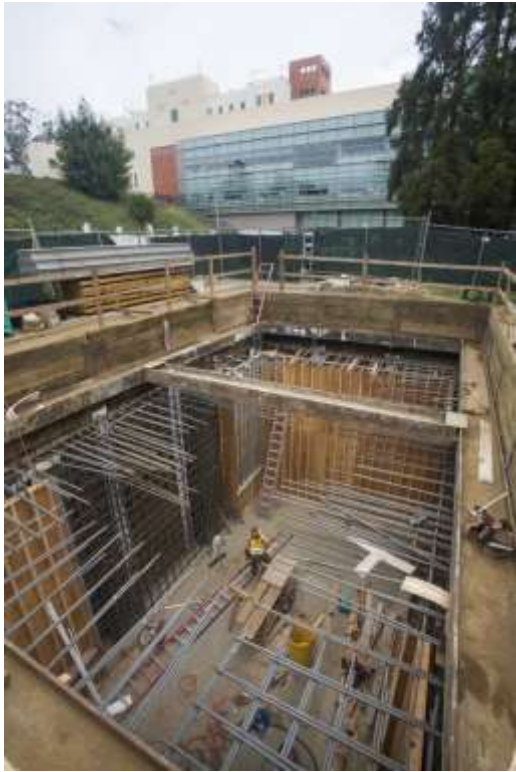
Laguna Honda Hospital cistern
