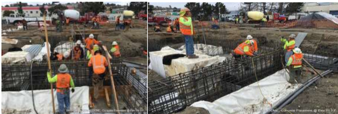
Service Elevator pit concrete slab
