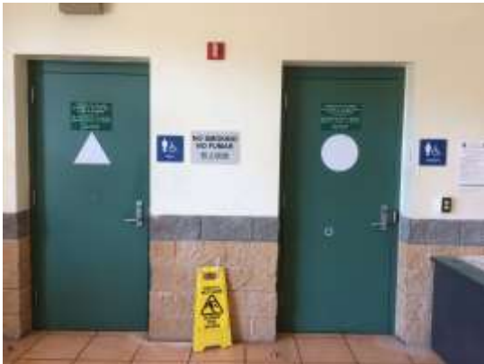
Mission station: new door and wall signage in ADA restrooms
