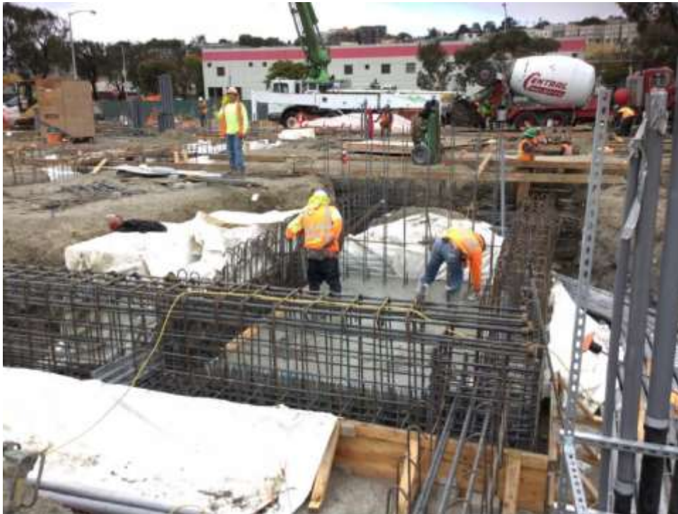
Placement of concrete slab at elevator pit
