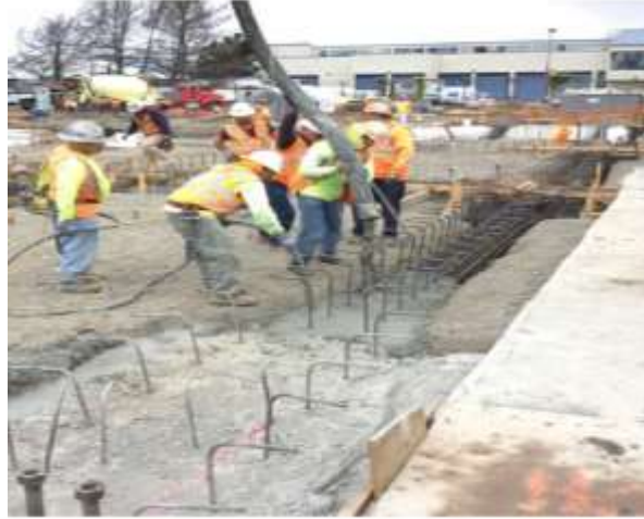
PC's & GB's concrete placement
