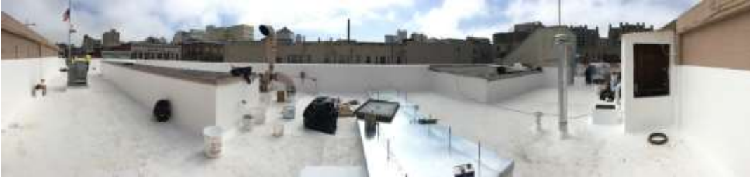
FS 3 Roof, HVAC and Generator Replacement – under construction
