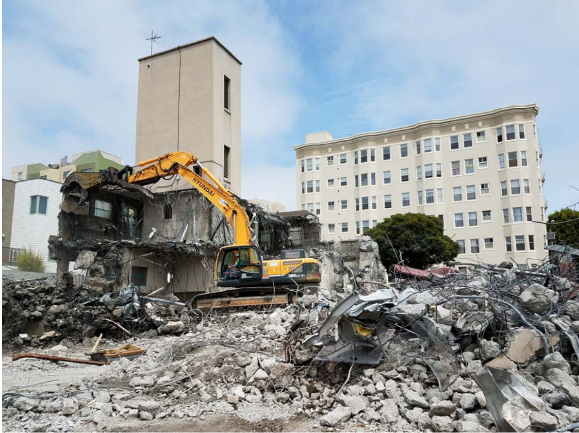
Fire Station 5 – Building Demolition (May 30, 2017)
