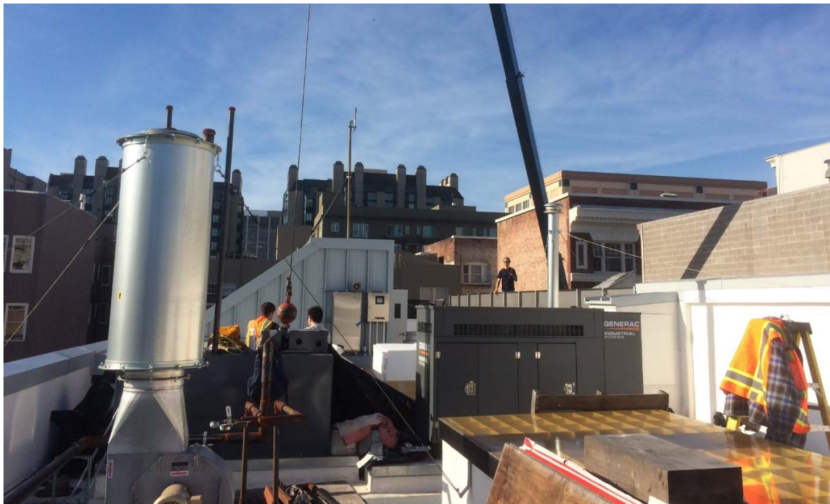
FS 3 Roofing, HVAC, and Generator Replacement
