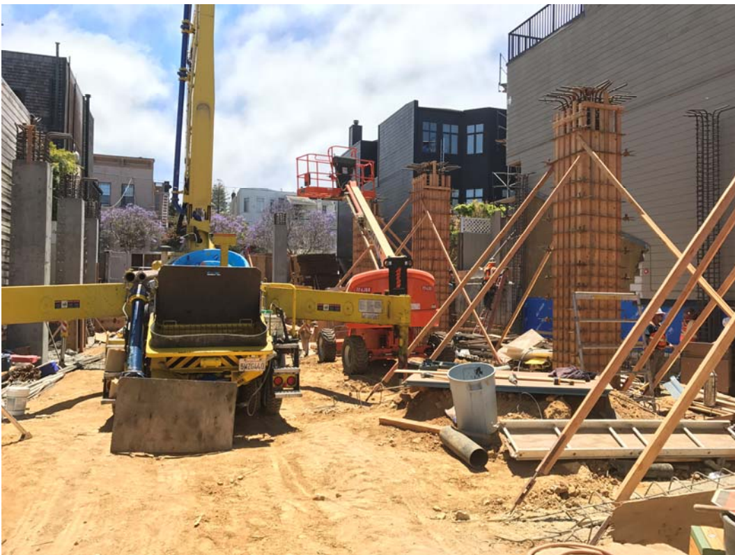
Fire Station 16 – 1st Floor Columns Concrete Pour (June 29, 2017)
