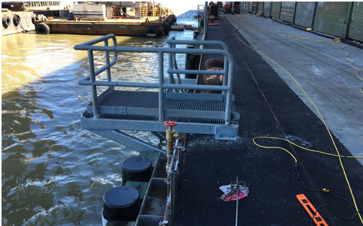
Pier 26 Fire Boat Berths – under construction
