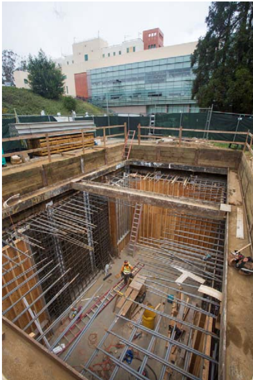
Laguna Honda Hospital cistern
