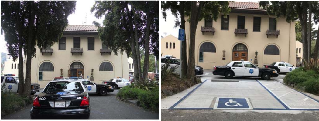
Park Police Station – Before and after photos of new accessible parking space and signage.
