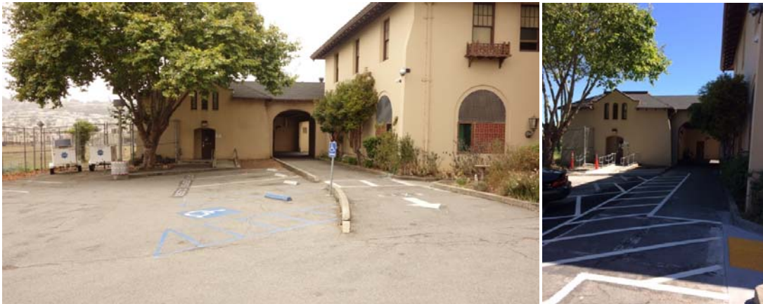
Ingleside Police Station – before and after photos of new accessible path of travel on site.
