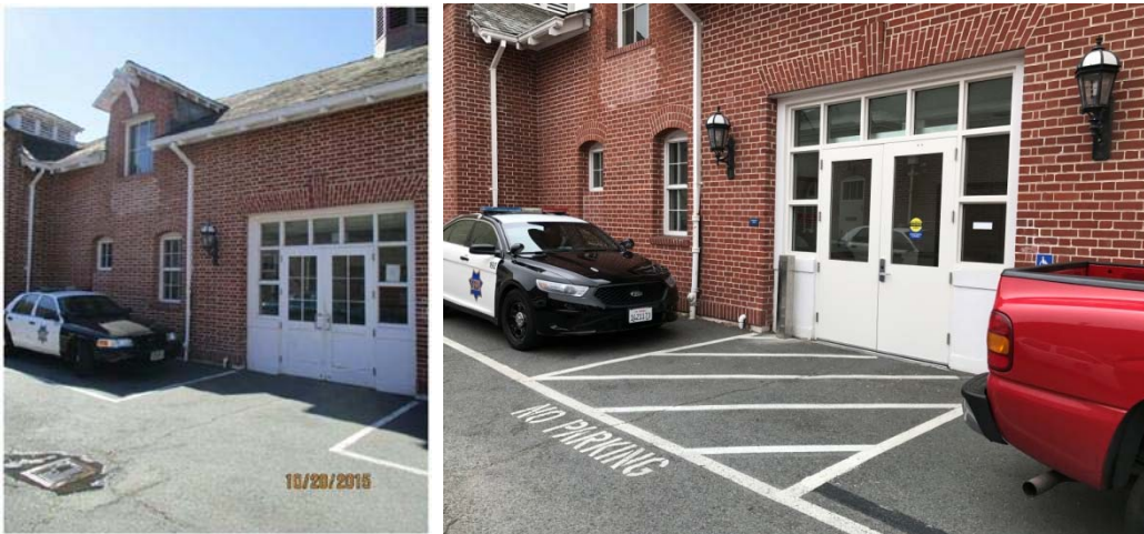
Richmond Police Station – Before and after photos of striped paths in front of community room with new accessible door hardware.
