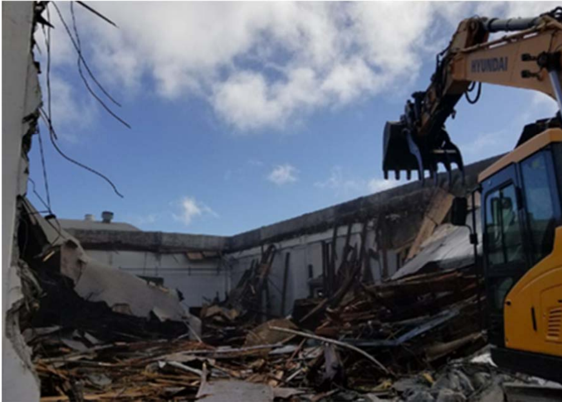
Demolition of Existing Bakery (May 9, 2018)
