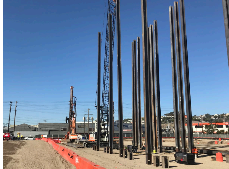
Drilling Deep Foundation Steel-H Piles into Bedrock – November 1, 2019
