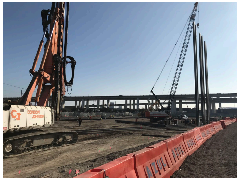
Drilling Deep Foundation Steel-H Piles into Bedrock – November 5, 2019
