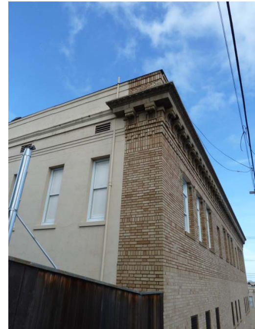
Existing rear facade
