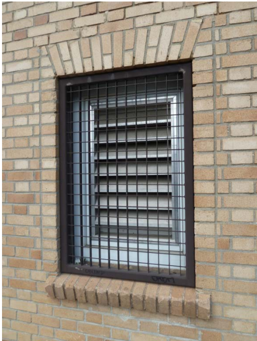
Existing brick pointing at windows
