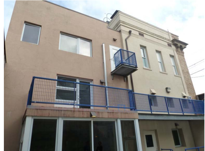
Existing rear facade
