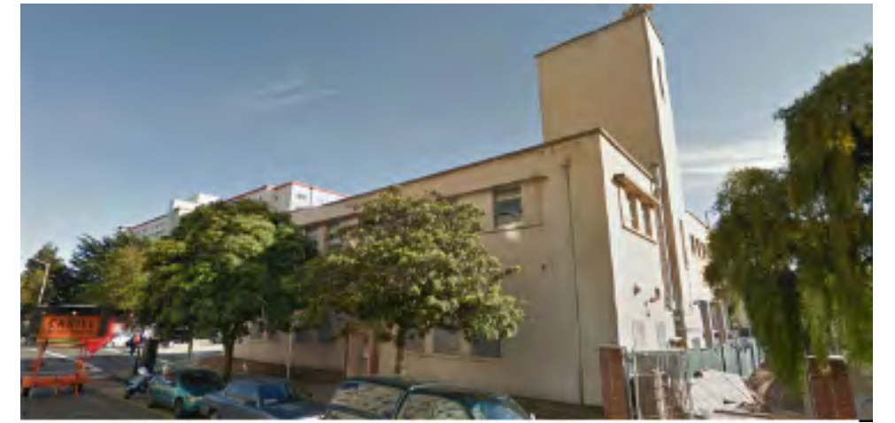
TURK STREET - NORTH & WEST FACADES
