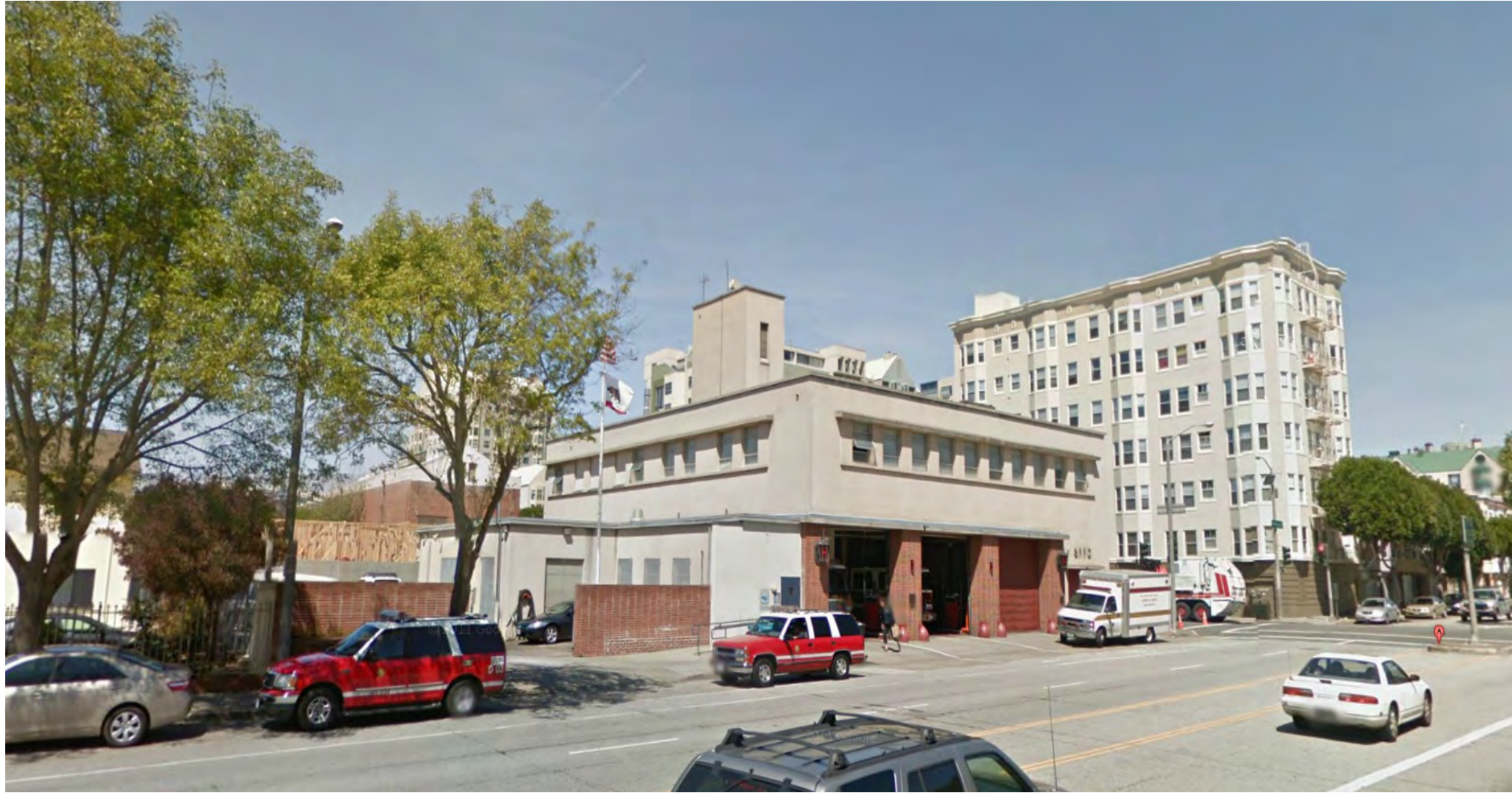
WEBSTER STREET - SOUTH & EAST FACADES
