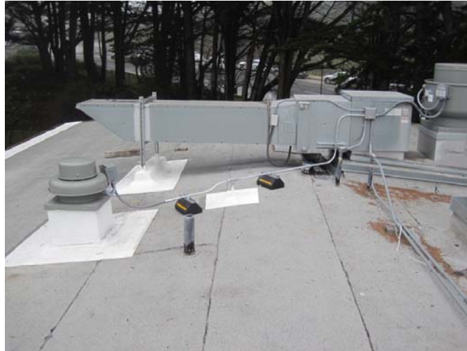
FS10 roof flashing @ mechanical unit
