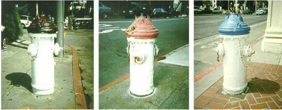
AWSS fire hydrants
