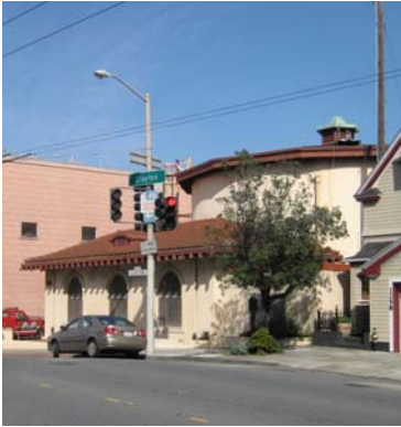
Ahsbury Heights Tank
