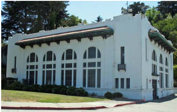
Pump Station No. 1
