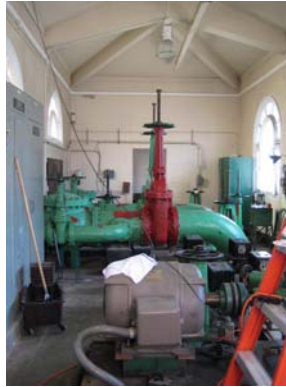
Gate Valve House Interior
