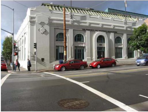
Pump Station No. 1
