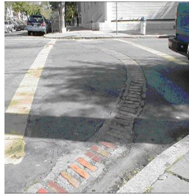
Exposed cistern perimeter brick
