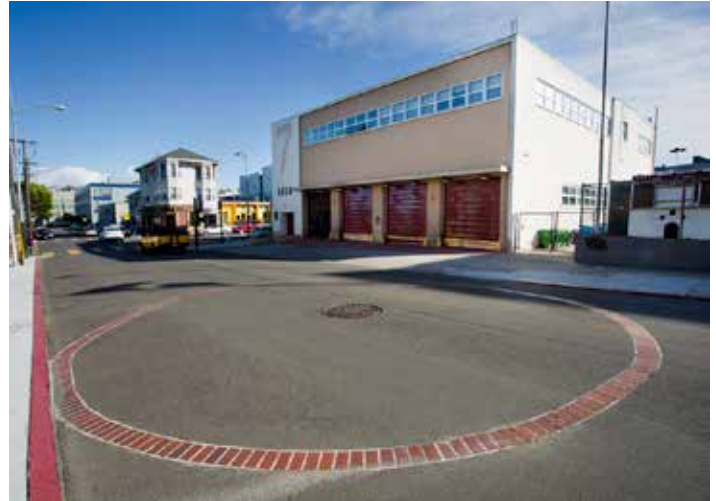
Brick ring indicating cistern below
