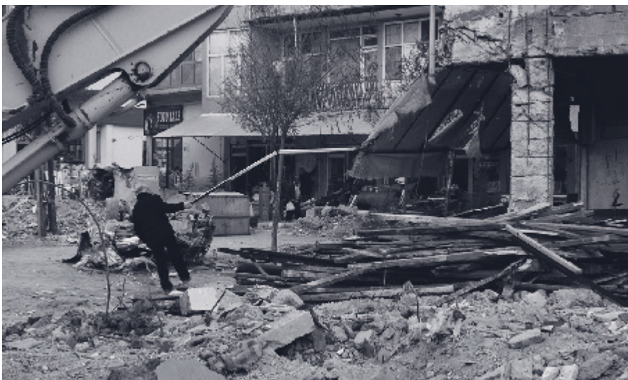
Damage from the 1989 Loma Prieta earthquake
