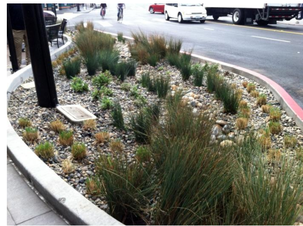
Biofiltration planters collect rain and recharge the watershed
