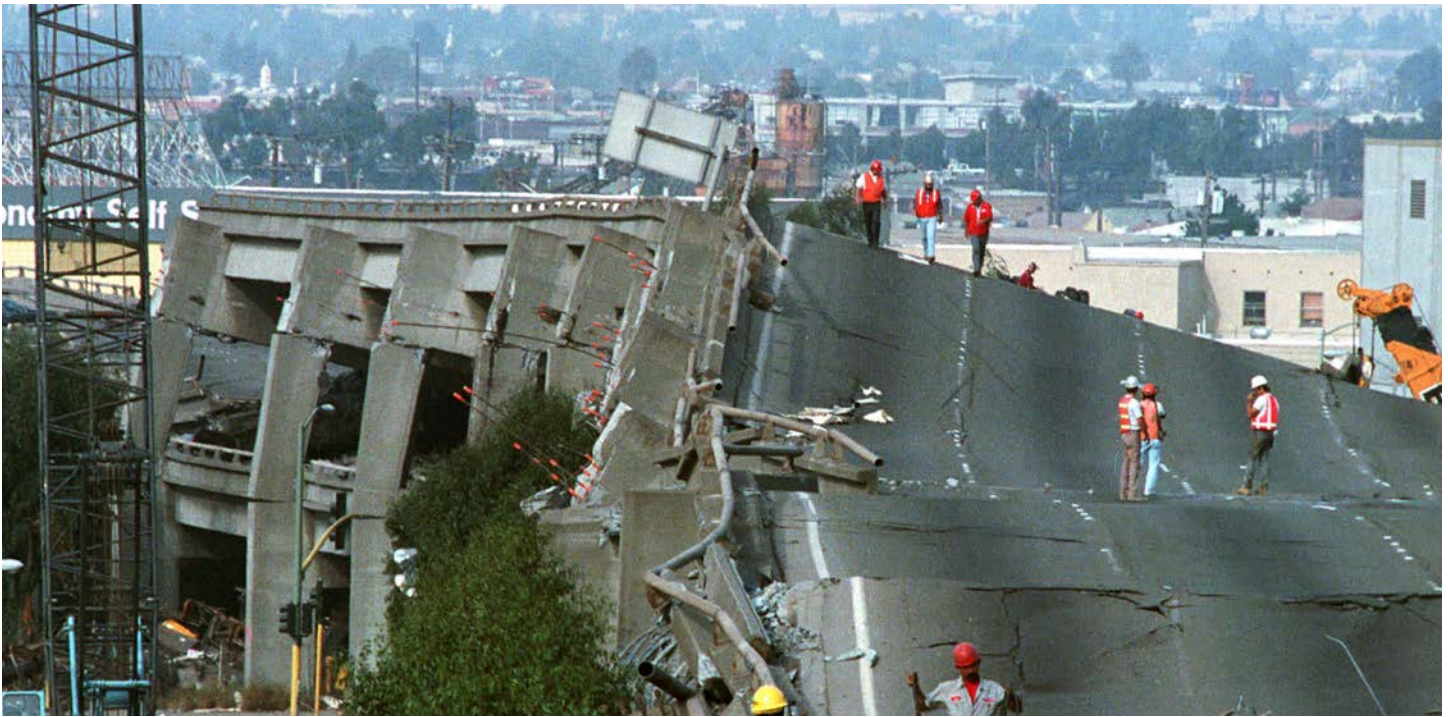
Aftermath of the 1989 Loma Prieta Earthquake.
