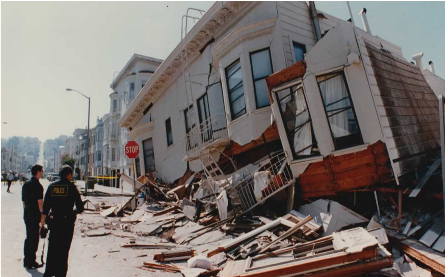
Aftermath of the 1989 Loma Prieta Earthquake.
