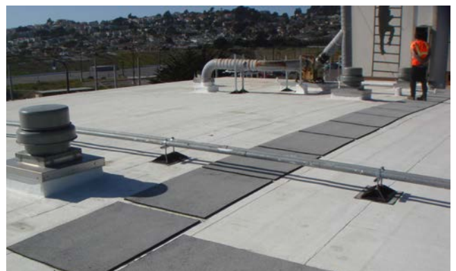
Fire Station No. 15: roof replacement (after)
