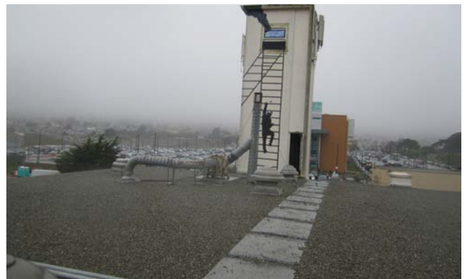
Fire Station No. 15: roof replacement (before)
