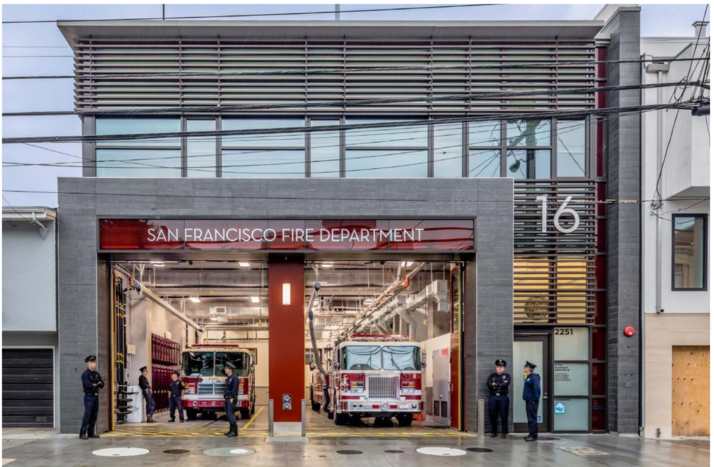
The new Fire Station No. 16 meets today's seismic safety standards.
