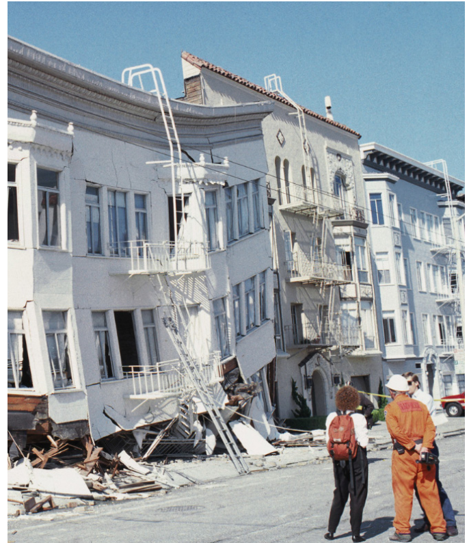
Aftermath of the 1989 Loma Prieta Earthquake.
