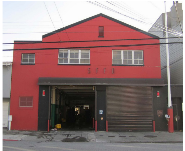
The old Fire Station No. 16, at 2251 Greenwich St. in Cow Hollow, was seismically vulnerable.
