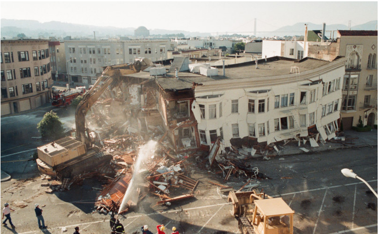
Aftermath of the 1989 Loma Prieta Earthquake.
