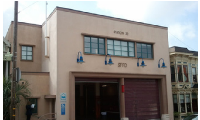
Fire Station No. 32: roofing, windows, exterior envelope and mechanical improvements
