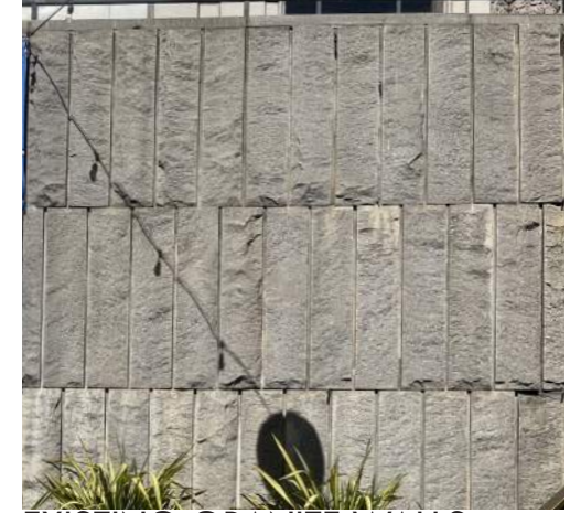
EXISTING GRANITE WALLS
