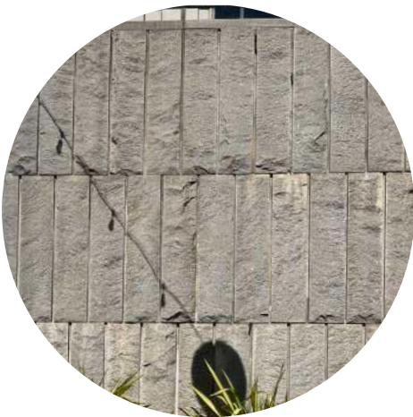
EXISTING GRANITE WALLS
