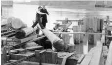
Third Street Sewer
