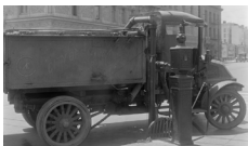
Catch basin cleaner at Eddy and Taylor Streets
