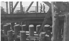
Third Street Bridge
