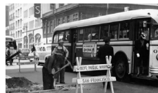
A repair crew works at Mission and Fourth streets.
