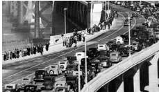
Bay Bridge opens.
