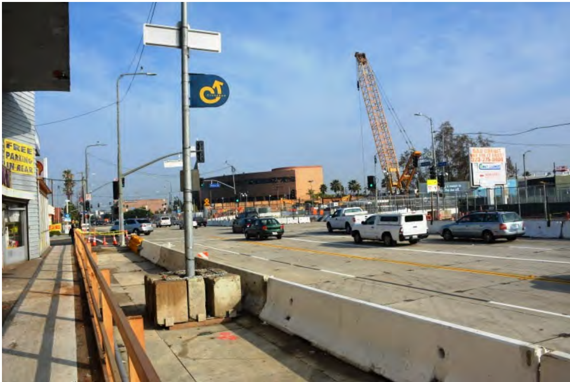
Figure MR-3. Photograph of Traffic Flow Over Decking While Excavation Continues Below
