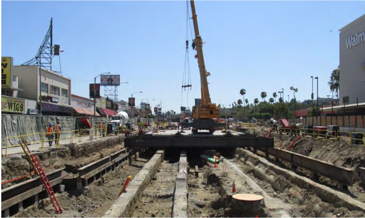
Figure MR-2. Photograph of Decking Installation
