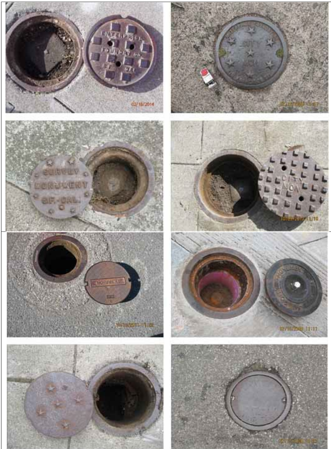
Some Typical Monuments with Well Casings
