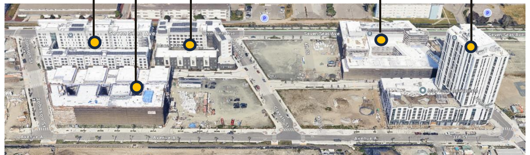
Public Infrastructure + 5 Buildings Complete (653 Units) 2024
