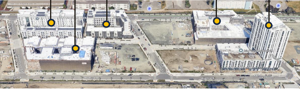
Public Infrastructure + 5 Buildings Complete (653 Units) 2024
