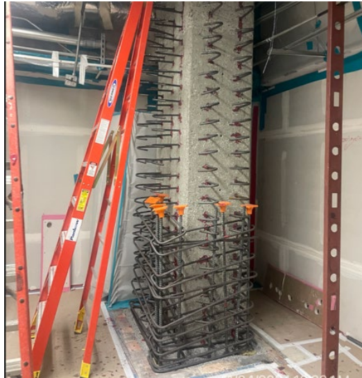
Existing Concrete Column Enlargement
