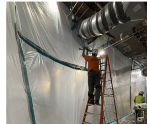
Typical IC barrier setup
