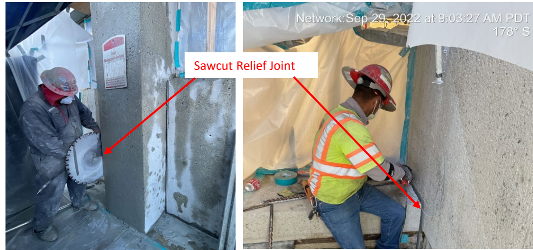
Exterior beam spandrel sawcut and caulking
