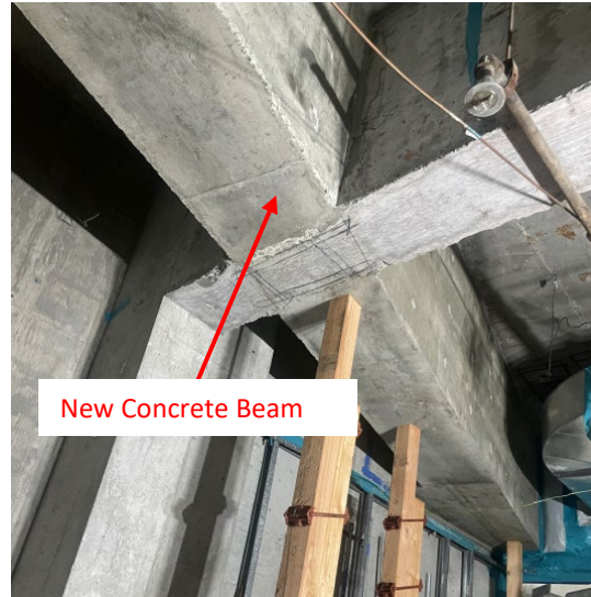
Added Concrete Beams
