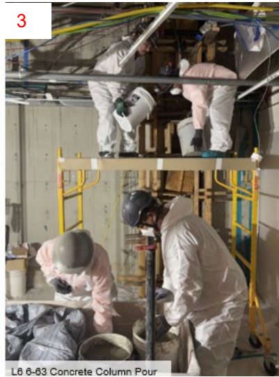
Photos #1-4: Construct new steel beam and column and new concrete column
