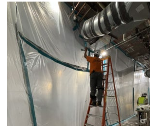
Typical IC barrier setup
