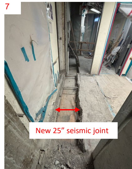
Photos #6-7: Chip out existing column and slab to create new seismic joint
