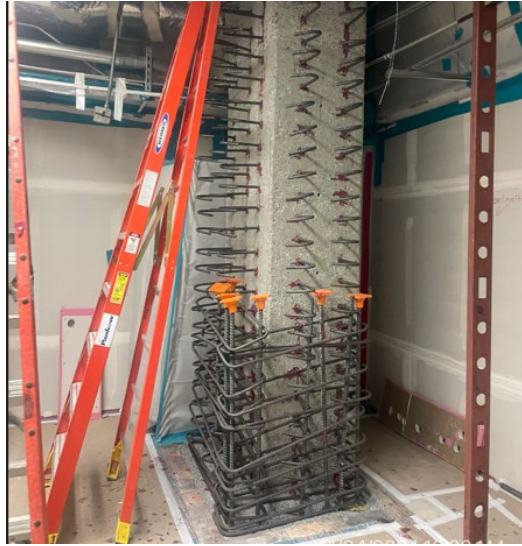
Existing Concrete Column Enlargement
