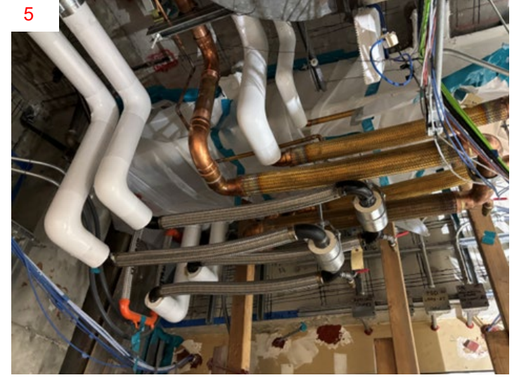
Photo #5: Install new flexible connections for all existing utilities
