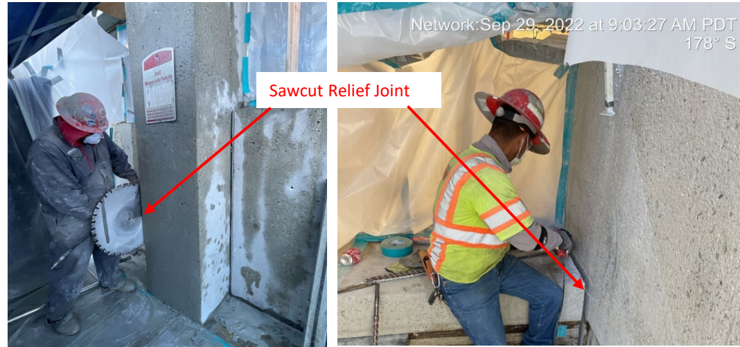
Exterior beam spandrel sawcut and caulking
