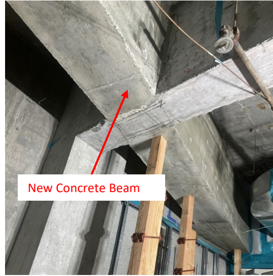
Added Concrete Beams
